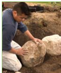
14 Build retaining wall
