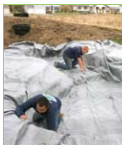
6 Install liner and underlayment
